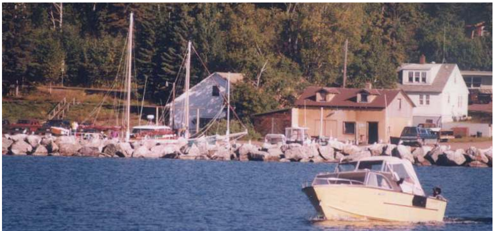
Below: The Yellow House (right) before it was yellow. Prior to being purchased by North House, the building was owned by the Eckel family of Grand Marais.
